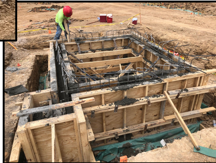
Grade Beams and Elevator Pit
